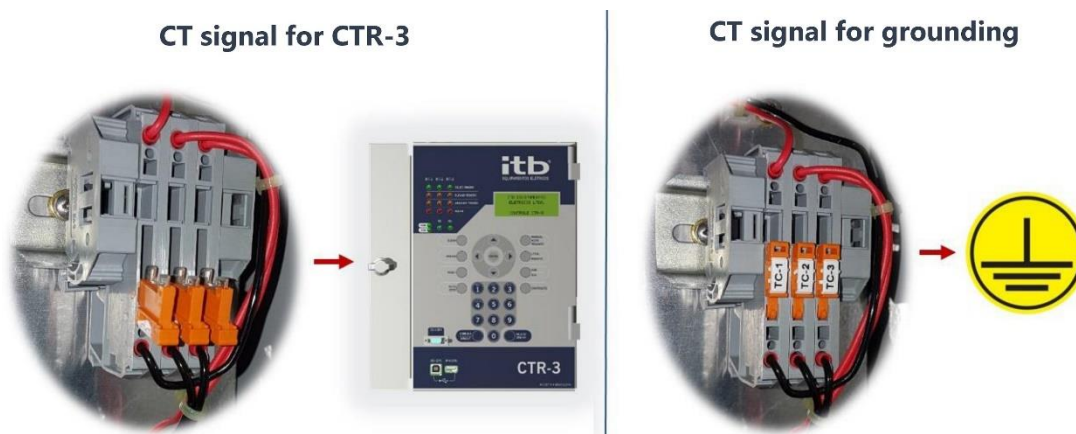
Figure 6: Procedure to short circuit the CTs.
